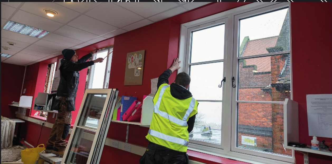
On-going project - Centurion Windows Carefully fitting R9 into Scarborough College.
